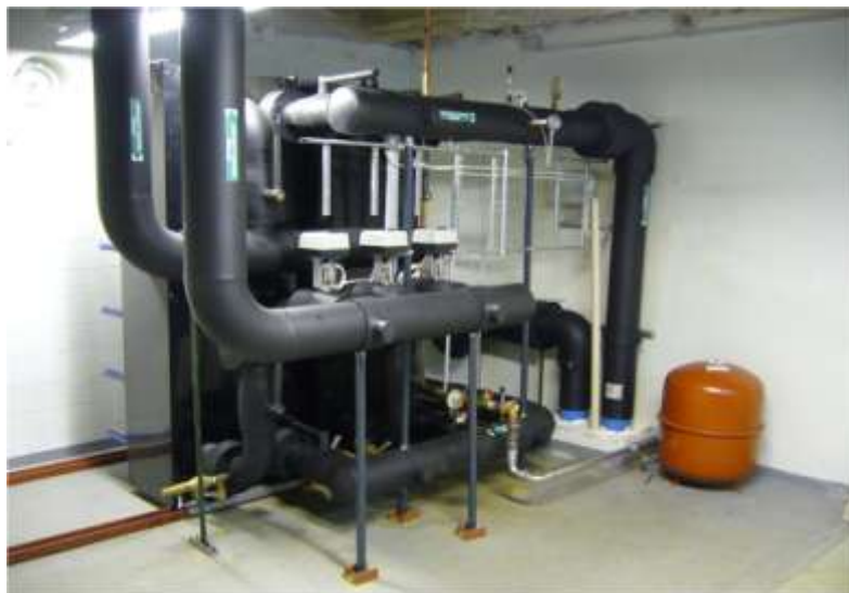
Figure 1: A DC substation with heat exchangers and expansion tank (Source: HELEN Ltd.)
