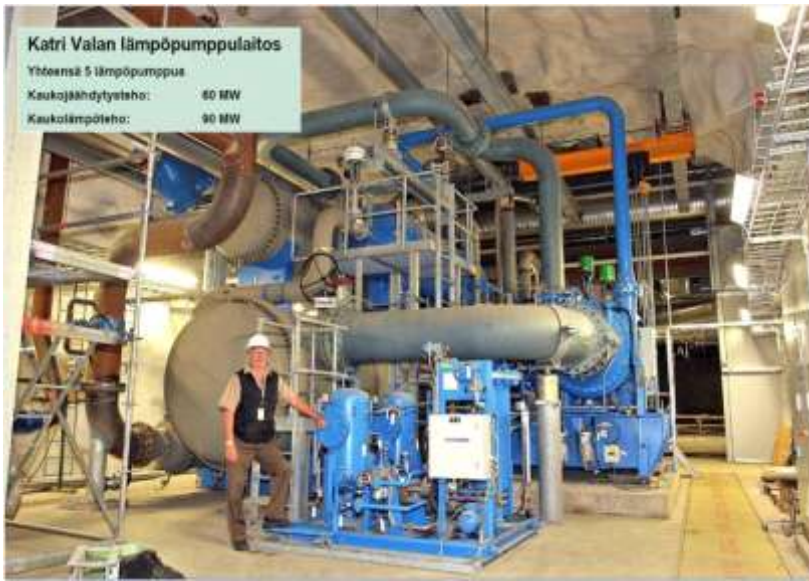
Figure 9: Katri Vala HP plant in Helsinki for combined DHC with five heat pumps for heating (60 MW) and cooling (90 MW) as the largest of its kind in the world, awarded as best practice by the International Energy Agency (IEA) and the Euroheat & Power in 2009. (Source: HELEN)
